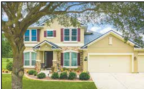
429 Buckhead, St. Johns 5 Bedroom, 3.5 Bath 3484 sq.ft • $959,900 Screened Pool Home (CBC) overlooking lake preserve. First floor ownwrs suite.
