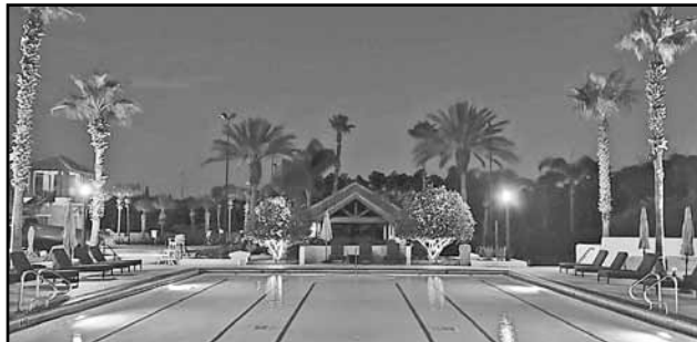
Above, additional lighting has been added to the pool deck.
