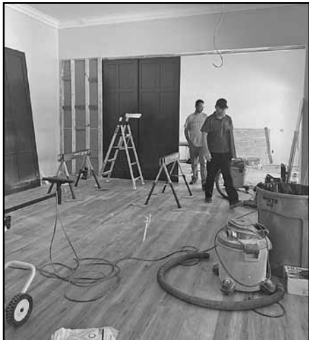
Workers install new flooring at Amenity Center.
