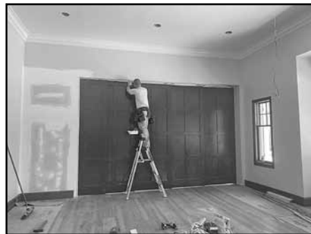
Installing tall pocket doors to divide the Lounge from the Gathering Space.
