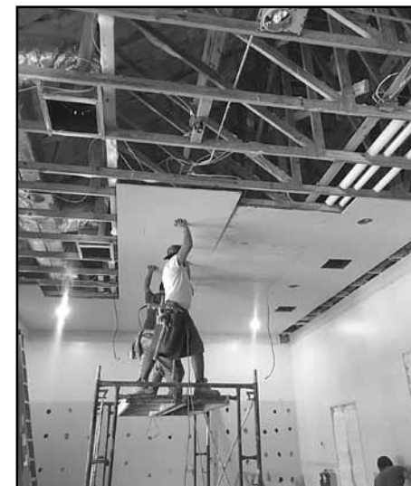
Raising the ceiling at the Amenity Center
