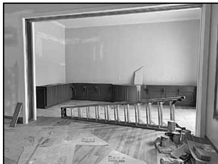
Installing tall pocket doors to divide the Lounge from the Gathering Space.
